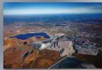
The treatment area at LKAB's Kiruna mine, with water treatment tanks and settling.
