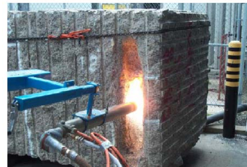
Figure 20. Plasma torch applied in a vertical sweeping motion.
